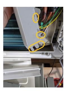
5.) Locate the coil mounting screw on the right side of the coil, in front of the motor housing (highlighted in yellow). Remove and reinstall loosely (4 turns from tight.)
